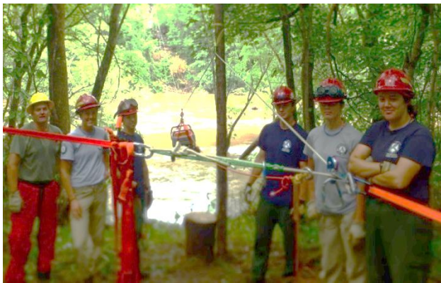
Generator evacuation across flooded St. Francis River, Silver Mines Rec Area gating project.
