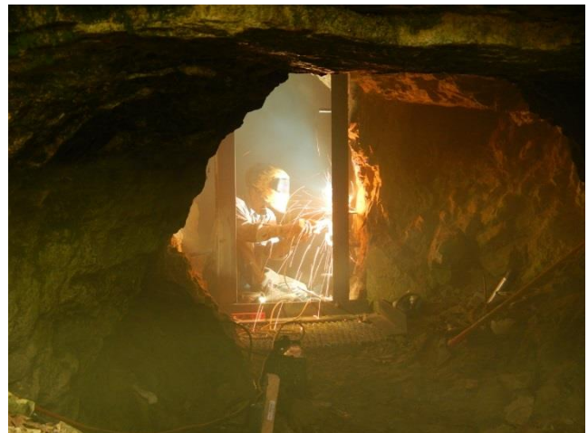
Dennis Novicky welding up the last (Butler Hollow Mine) gate.
